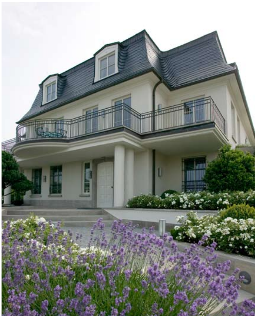
← Family home Built with: MULTIPACT® advance // Photo: ISOLAR®
